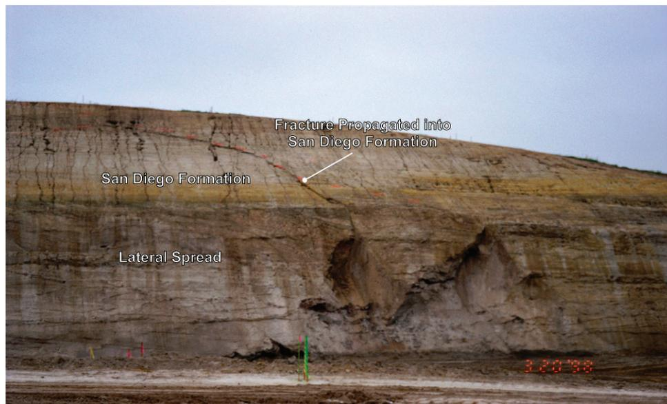
Figure 14. Photograph of a construction failure in progress. The fracture propagated up into the San Diego Formation from the Otay Mesa Lateral Spread, requiring large amounts of additional earthwork and stabilization efforts.
