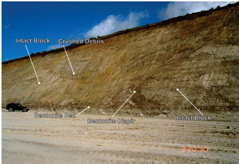
Figure 5. Photograph of a portion of a butress back cut along Poggi Canyon, west of Figure 4. Note the intact blocks of sandstone separated by the bentonite diapir and zone of disturbed sandstone, siltstone, and claystone. The horizontal bentonite bed on which the Otay Mesa Lateral Spread failed is clearly visible.
