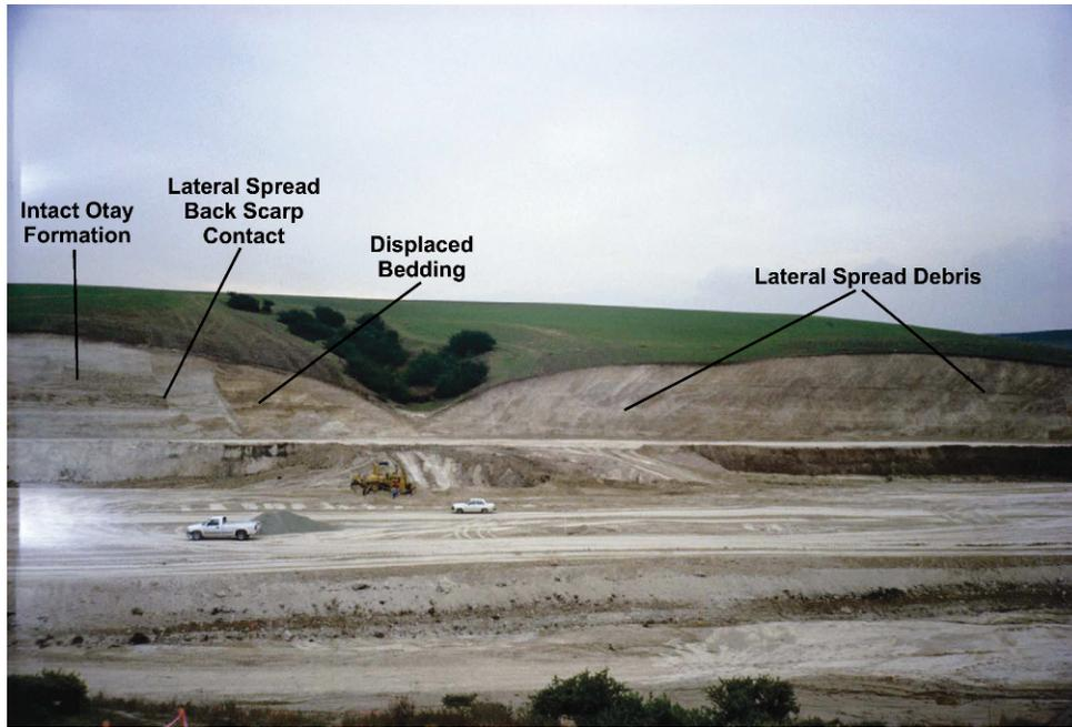
Figure 4. Photograph of a portion of a butress back-cut slope along Poggi Canyon, looking south. Note the back scarp contact between the intact Otay Formation and the Otay Mesa Lateral Spread deposit, and the backward-rotated bedding. Of particular interest, note the lack of topographic expression of this contact.
