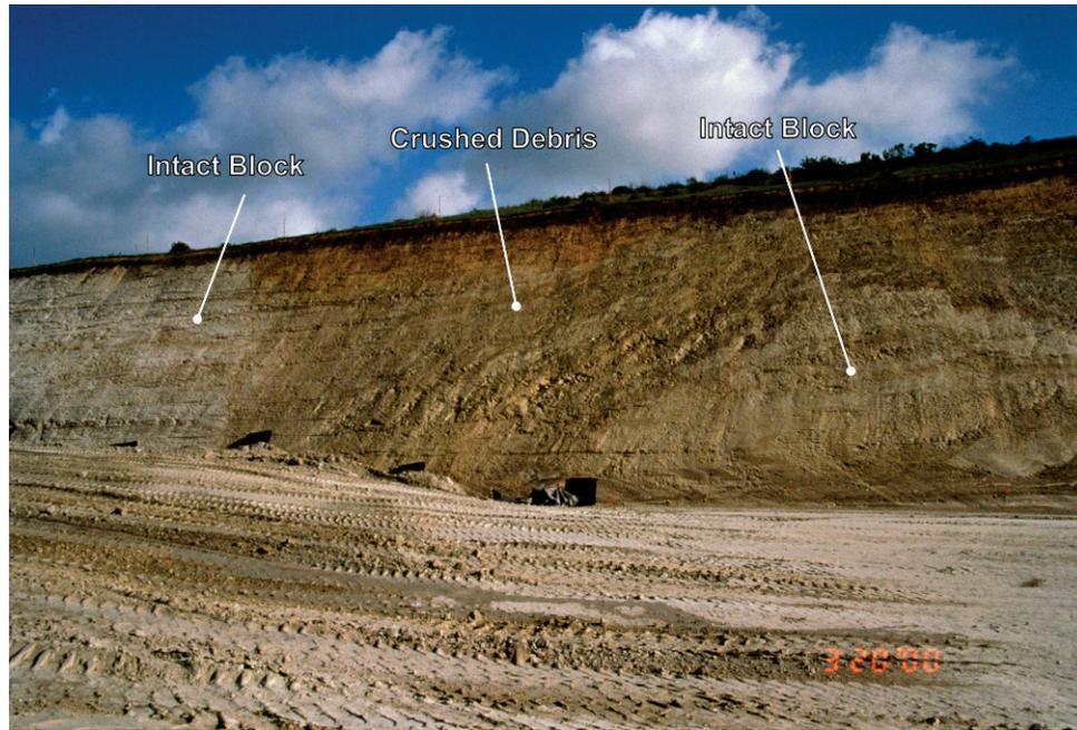
Figure 6. Photograph of a portion of a buttress back cut along the south side of Poggi Canyon east of Figure 5. Note the sheared and fractured debris zone. The reddish, oxide-stained area at the top of the cut in the fractured debris is often mistaken for San Diego Formation. As a result, the north-south-striking contact between the fractured and unfractured debris can be misidentified as a trace of the La Nacion fault.
